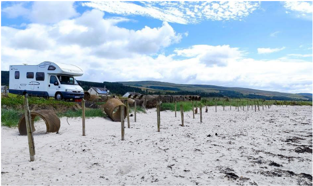
Figure 13. Fencing and old concrete pipes are struggling to consolidate sand built up here since the 1960s adjacent to the Tayinloan ferry terminal.
