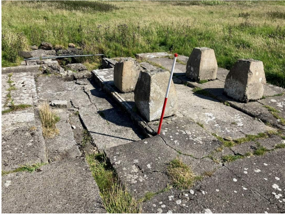
Figure 46. Foundations of steam engine used to power radio station (SCAPE ID: 16832)
